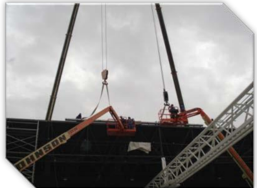
Mobilization on Site
